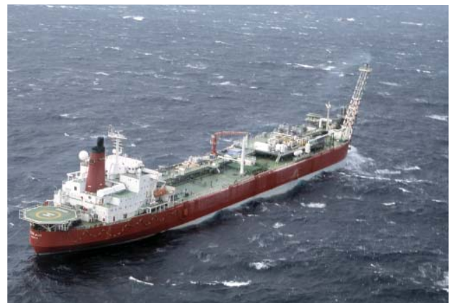
Figure 1 ■ FPSO Ikdam, Oudna field
